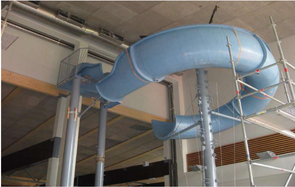
Picture: Water slide installation, Keuruu public swimming pool
